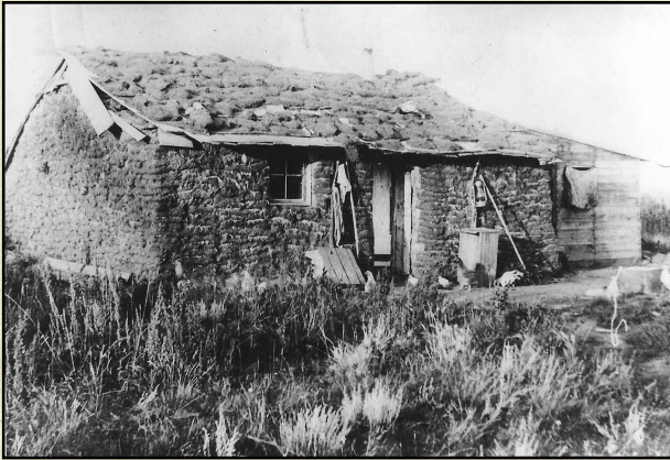
A soddy was a type of home built from sod (blocks of grass and soil) that was common on the prairies of Western Canada in the early 1900s. These homes were a practical solution for settlers who faced limited access to traditional building materials like wood or stone in the vast open grasslands.
